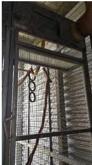
Figure 8: Closed external access door (all cages)
