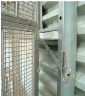
Fig 5: Locking bar mechanism
