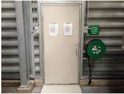
Fig.29 Outside access door
