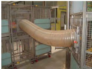
Fig 4: Transfer tunnel between PHU &amp; Flexagon
