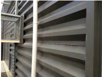
Fig.30 The external side of the building.
